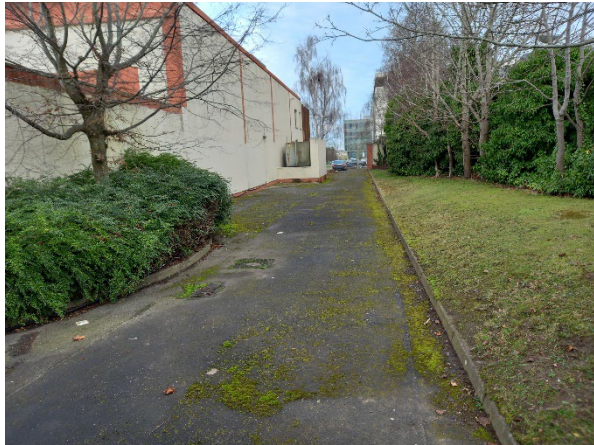
A7. View from the southern end of laneway at centre of site.
