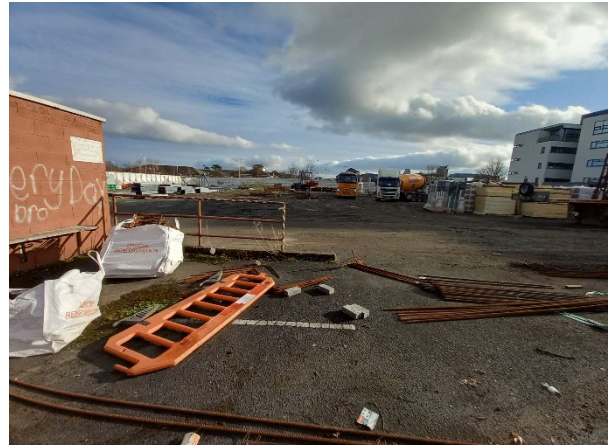
A8. Eastern section of the site showing active construction processes underway.
